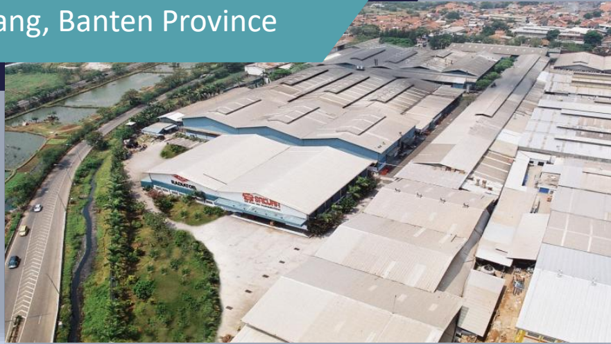
Kapuk Plant (Heat Exchange)
